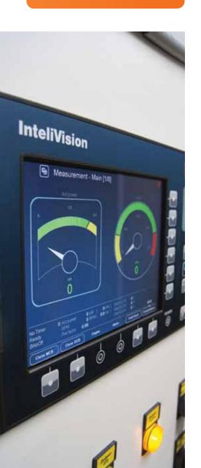
nontrol System manages all enreeniring system and auxiliaries of cogeneration heat power plant. To fullfill this function the specialist of Rolt Engeeniring elabourated control panel.
