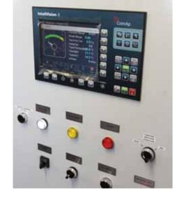
perator of power plant uses the control display which is on the front side of the auxiliaries cabinet and can set the following modes of operation:
