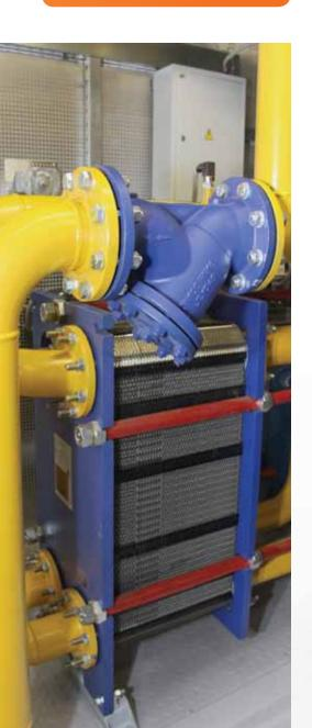
Payback period of the investments in autonomous power center depends on effective use of fuel (trunk gas, oil associated gas or diesel). It is a fact that during generation chemical energy of hydrocarbon fuel is modified to electric one with efficiency of 27-45% depending on generating equipment and its manufacturer. Remaining energy turns to heat which can be useful.
